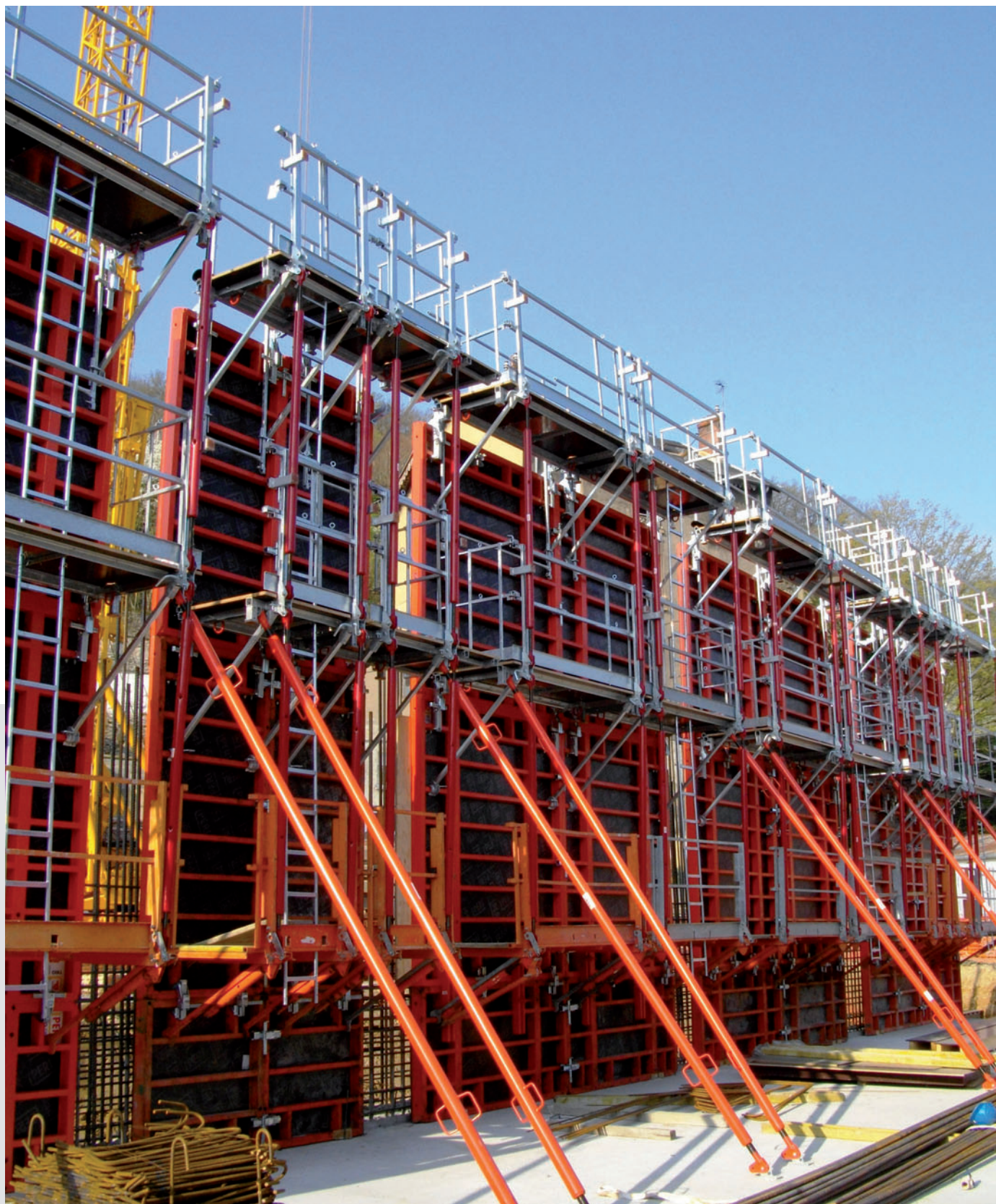
6.60 m high MAXIMO complete with MXP platforms and ladder access.
