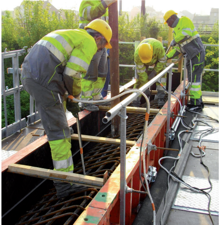
Safe working conditions on the MXP platform.
