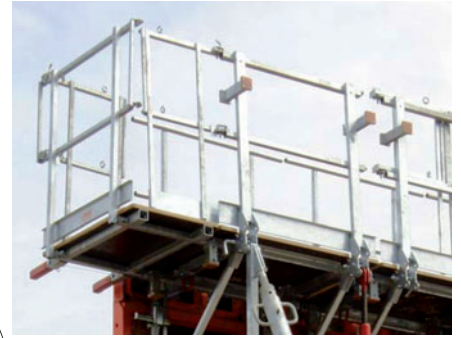
The MXP platform guardrails are simply folded downwards.
