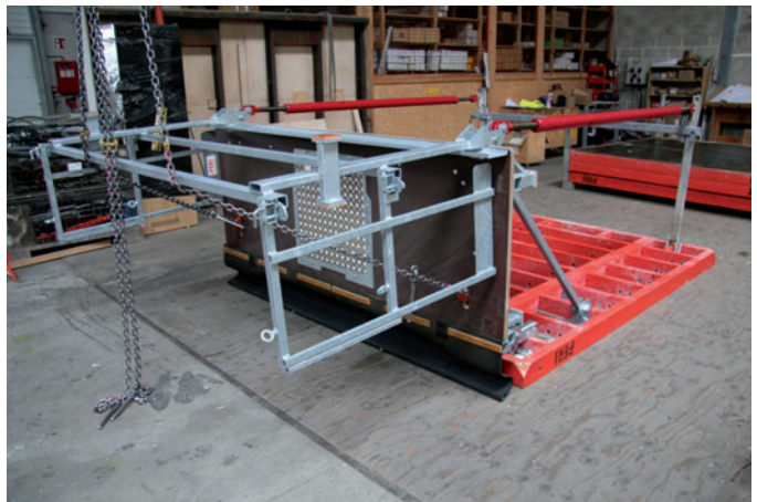
6. Mount push-pull props and horizontal struts.
