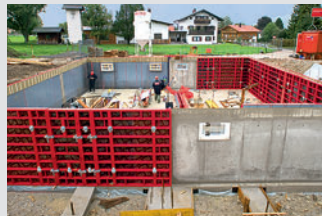
Wall Formwork
